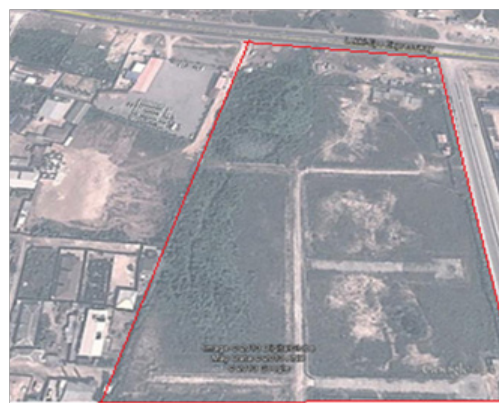
Figure 1 Aerial photograph of site and adjoining catchment areas.
