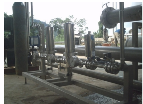
Plate 4.3. Cylindrical Container and Meter for the Treatment Plan
